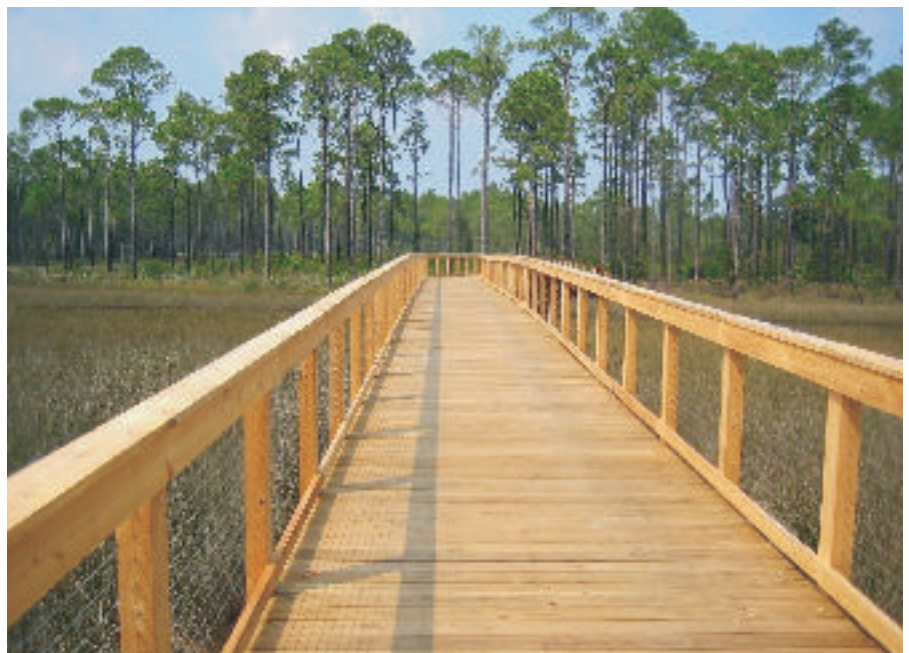
Wooden bridge at River Camp by St. Joe in Panama City, Florida using stainless steel cable.
